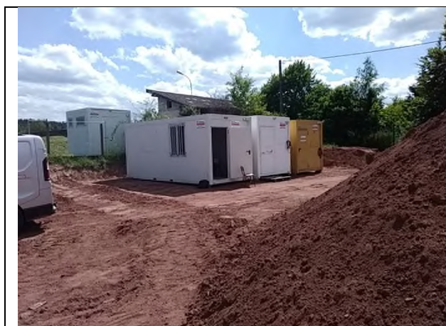
Installation base vie
